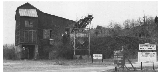
Workhouse Stone Crusher [1985 HwTwp Cultural Survey]
