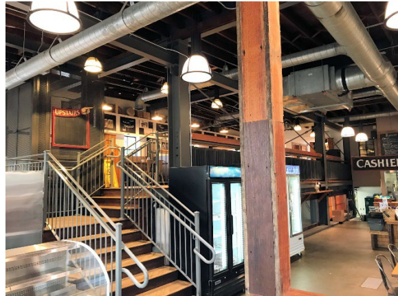
Brick Farm Market interior [DD 2023] Stairs up and windows to basement below
