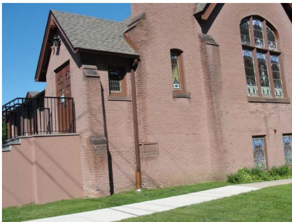
The southeast corner of the 1914 sanctuary, built of Hummelstown brick.
