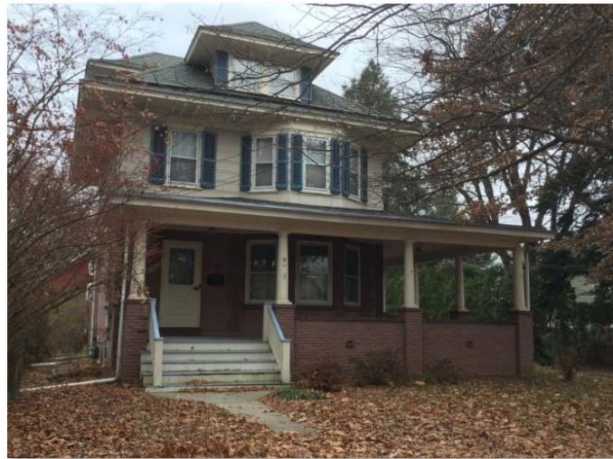
Number 9 Blackwell Avenue, with its porch foundation wall of Hummelstown Brick
