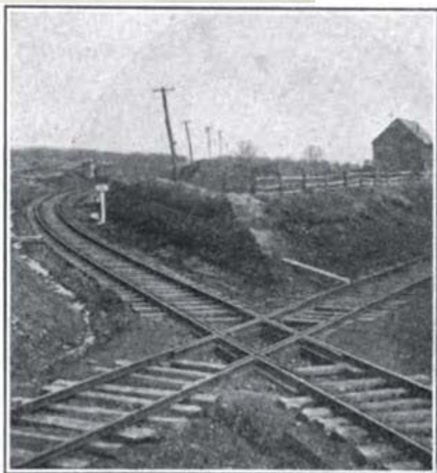
The Frog that Caused all the Trouble. From a Photograph Taken Shortly After the Battle.
